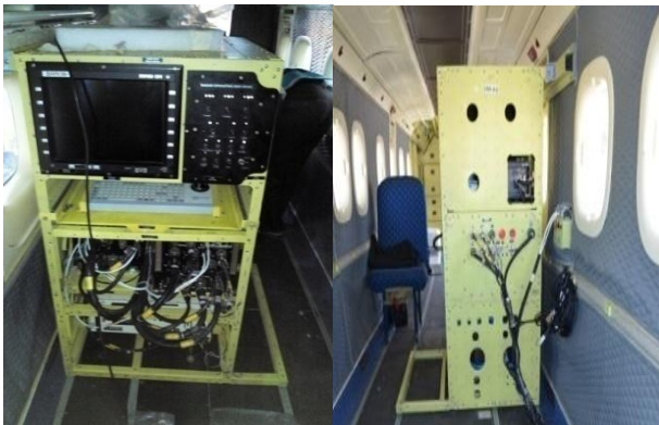
Figure 5 Installation of SAR Rack in FTB
